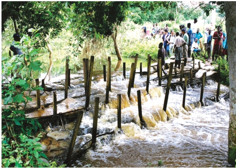
The use of local materials (soil and wooden) to construct weirs/dyks through farmers' self-support for affordability and sustainability is encouraged under Sawah
